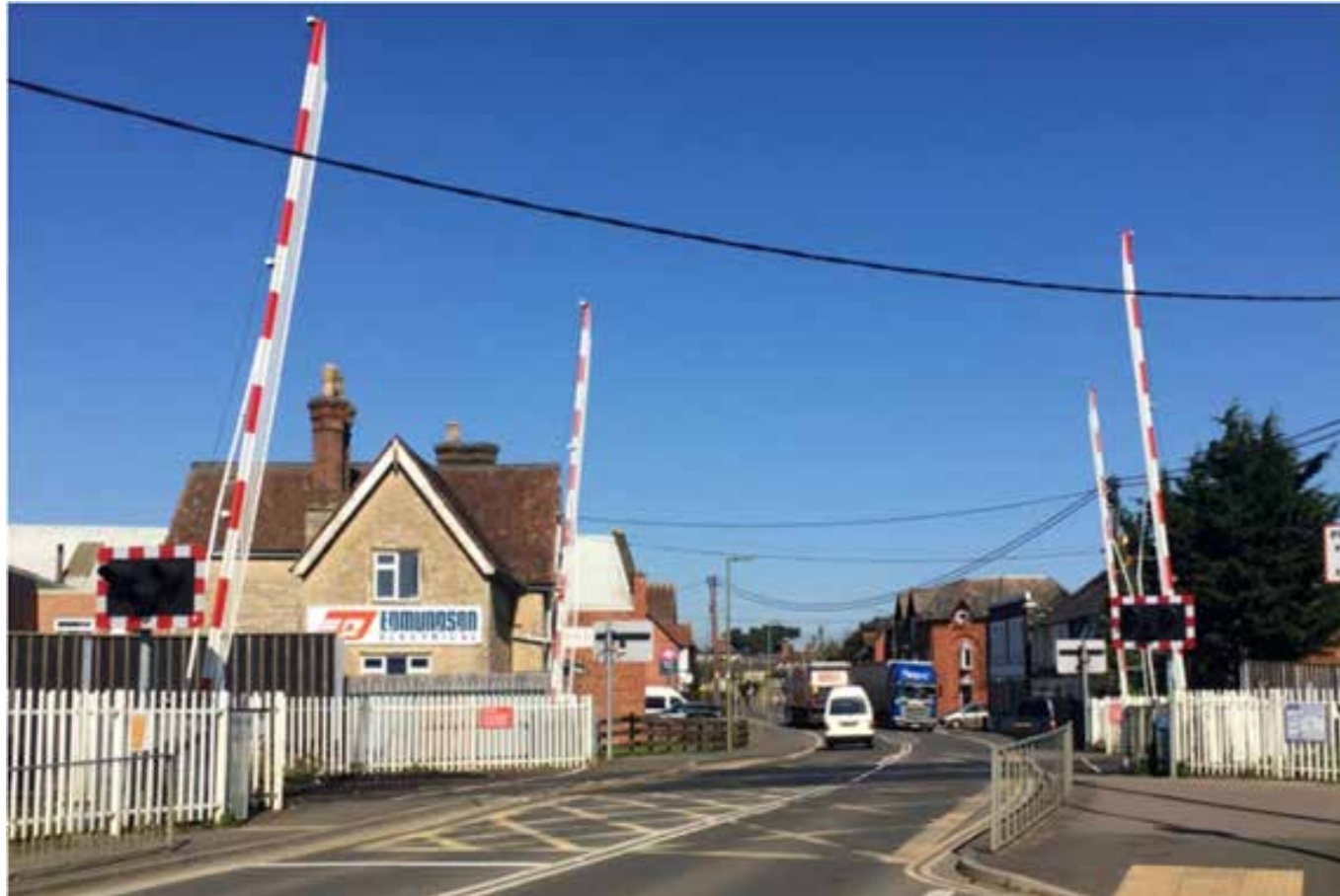
Figure 11: London Road level crossing
