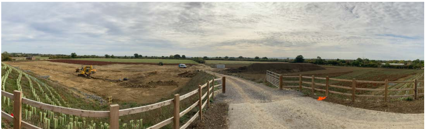
Land on the project currently in the process of being reinstated
