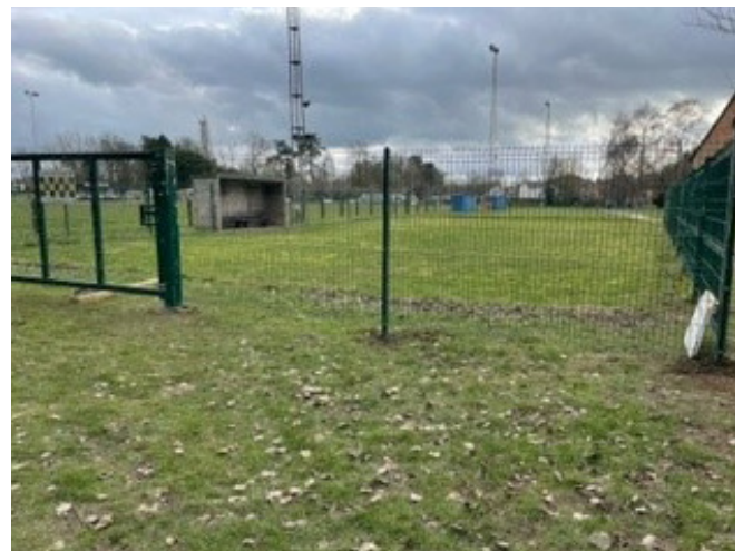
The Winslow Croquet Club with new fencing installed
