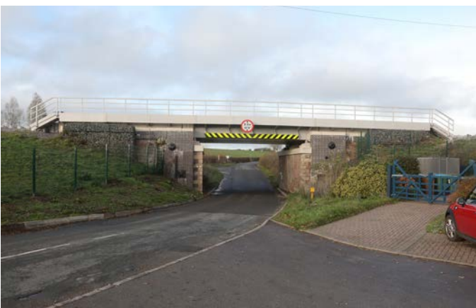
OXD32 Station Road Marsh Gibbon bridge
