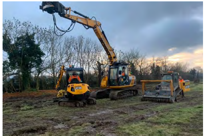
Wildside plant carrying out de-vegetation works.
